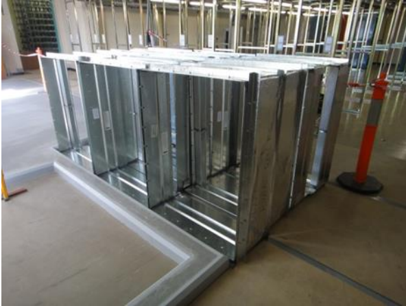
Insulation material fitted
