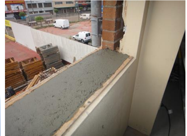
Bottom sill repaired prior to install
