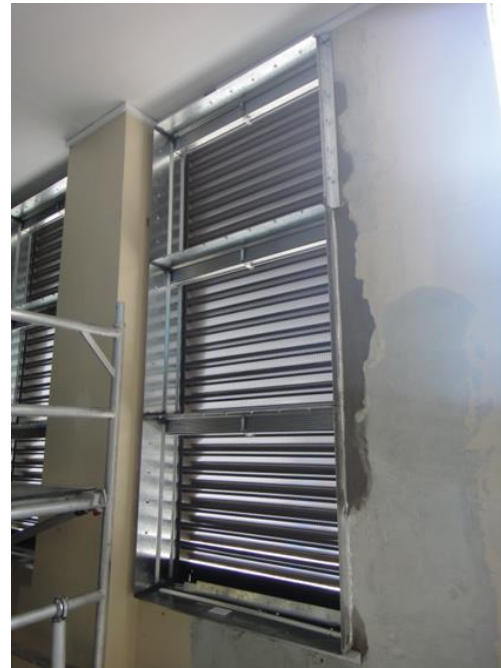
Dampers sections bolted together, edge of penetration repaired, angles being bolted on, twice the gap
