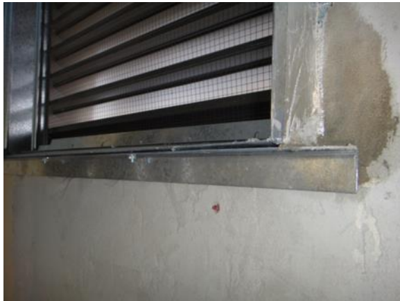
Insulation material fitted, angles being bolted on flush to wall
