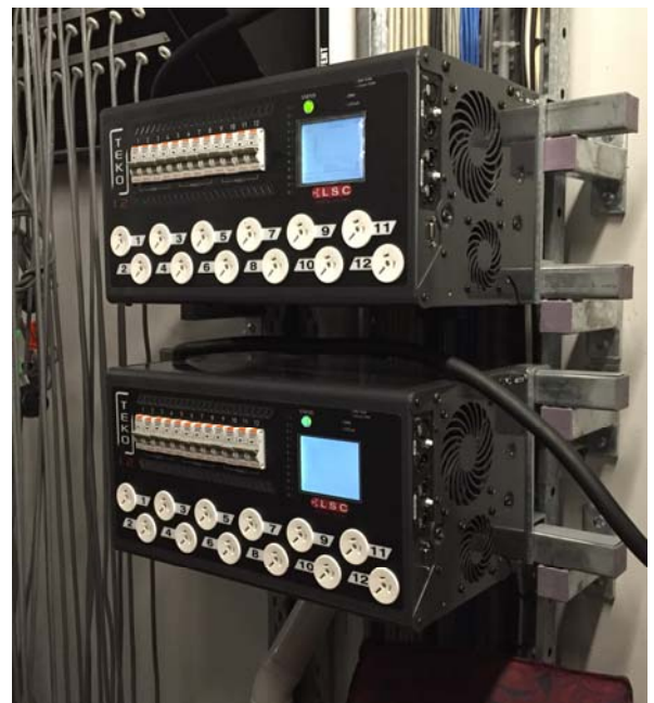
Two of the iTeko dimmers mounted on brackets.
