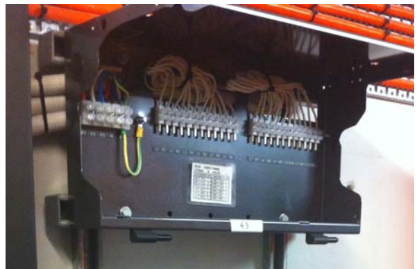
The iTeko clamshell frame that can be installed and wired prior to the dimmer arriving on site.
